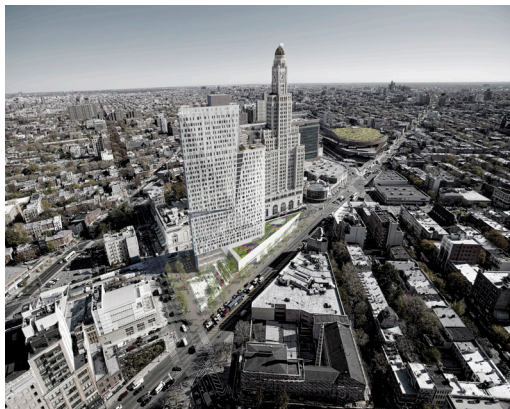
Aerial view of the future completed BAM South Tower.
