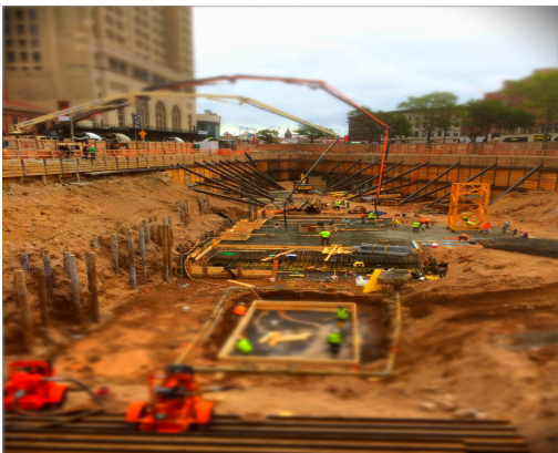
Over 6,000 yd 3 (4,587 m 3 ) of KIM treated concrete was used.
