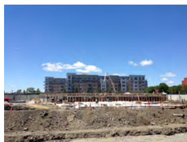
The KIM-treated foundations under construction
