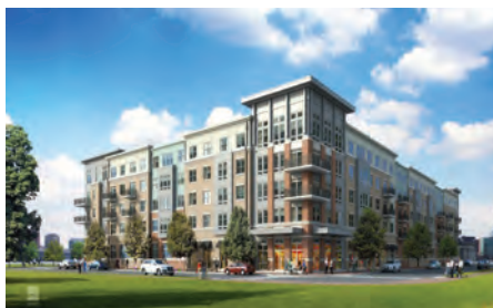
Kryton's concrete waterproofing system was able to protect against leaks, even with the building's position right on the waterfront.
